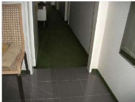
F: Entrance hall floor
