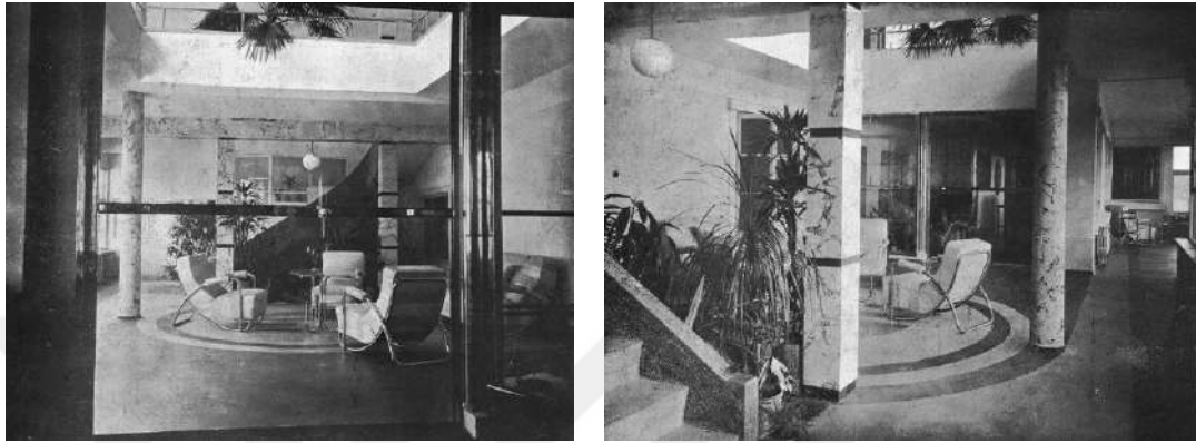
Figure 2.23. Üçler Apartment Block, a. , b. Interior view from the entrance lobby. Adapted from “Kira Evi: Ayazpaşa”, by S. Arkan, 1935, Arkitekt , 05, p.129-140.
