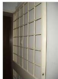
H: Entrance door
