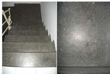
D, E: Stair Floor Material: Terrazzo
