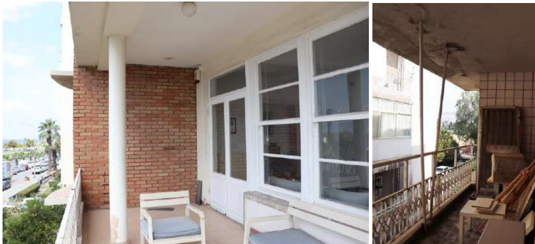
Figure 2.79. Paya Apartment Block, a. Original brick coating on the façade and wooden joinery, b. Steel V-Shaped columns on the balcony of the Paya Apartment Block
