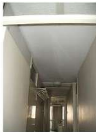
I: Entrance ceiling
