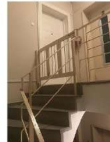
H: Railing Detail
