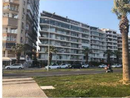
A: Çağlayan Apartment General View
