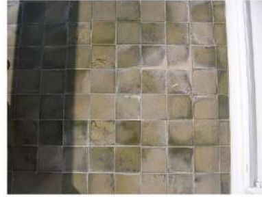
E: Balcony floor material
