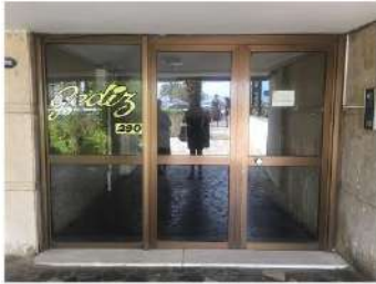
C, D: Apartment entrance door
