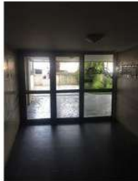
F, G: Entrance hall
