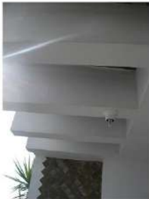
F: Balcony beams
