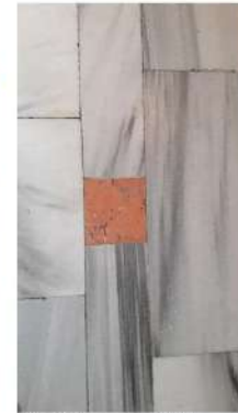
F: Entrance Hall Floor
