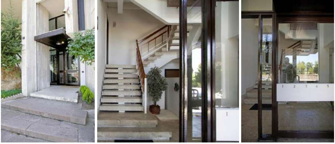
Figure 2.59. Çankaya Apartment Block, a. Entrance hall, b. Stairs, c. Entrance door. Adapted from Sivil Mimari Bellek Ankara 1930-1980, Retrieved from http://sivilmimaribellekankara.com/YapiDetayi.aspx?anah=279
