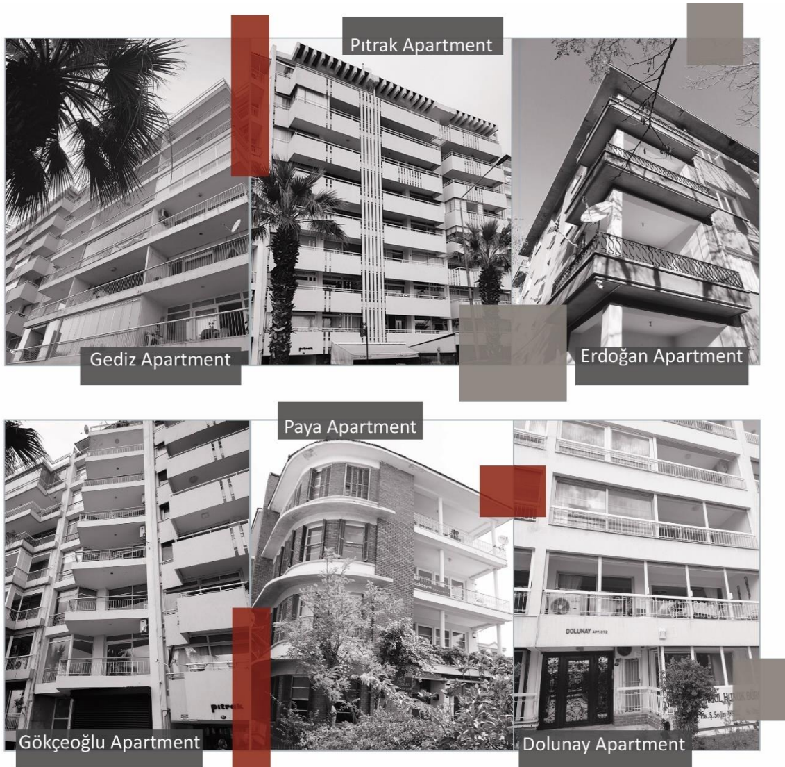
Figure 1. Selected Apartment Buildings from Karşıyaka, İzmir (designed by authors; photographs from authors' archives, 2016, 2019, 2020).
